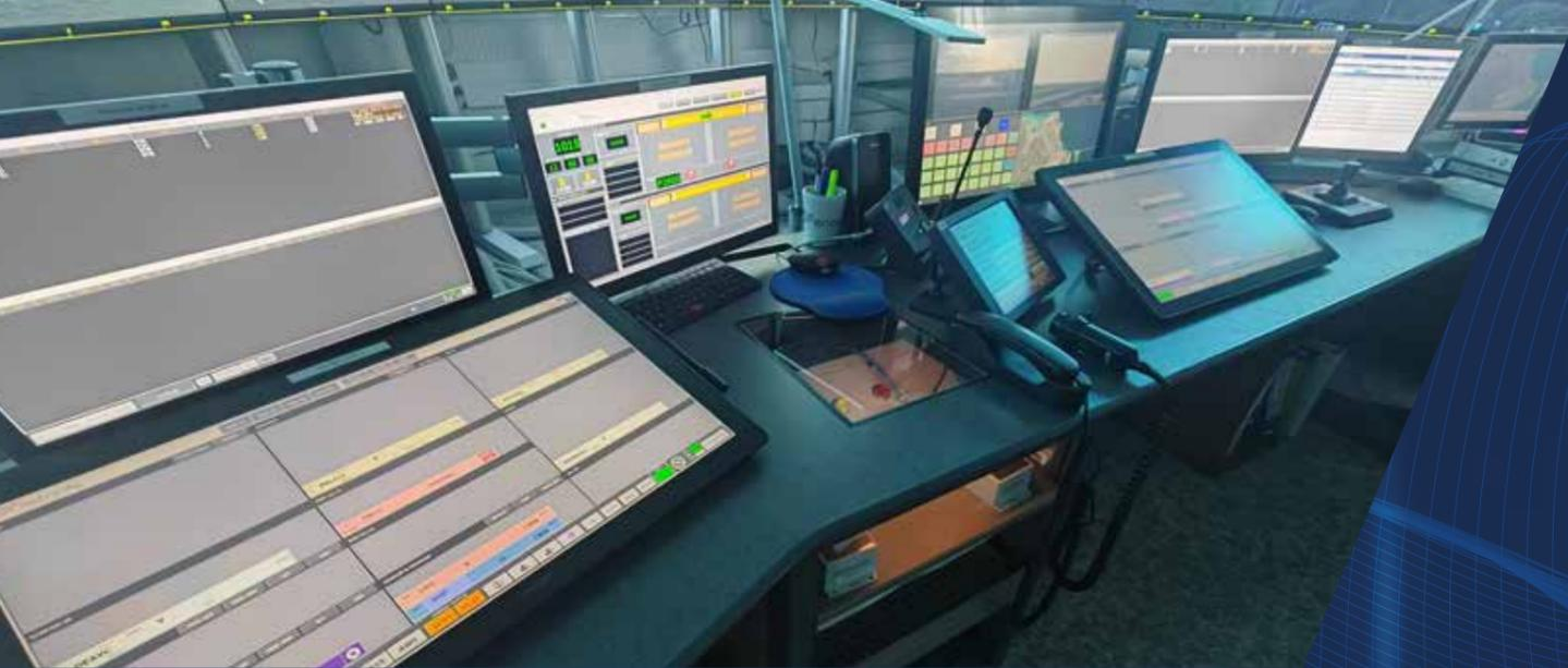
The introduction of remote digital towers represents an epoch-making revolution in the way airport traffic service is provided. The physical control tower is replaced by a digital operations room from which air traffic controllers can operate through the use of cameras and high-definition image monitors. The digital configuration improves the controller's situational awareness, thus offering operational and safety advantages.
